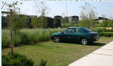
Parking engazonné (Nantes)
